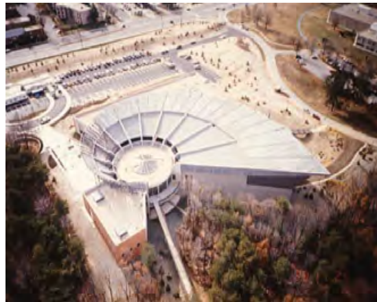
National Museum of the American Indian Collection Storage Facility, Suitland, MD
