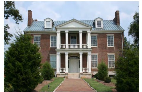
The Hermitage Restoration
